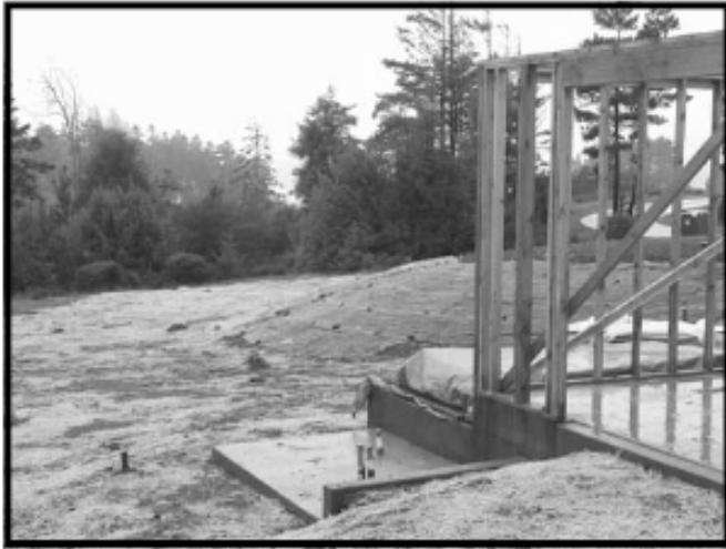
Controlling erosion protects water quality.
